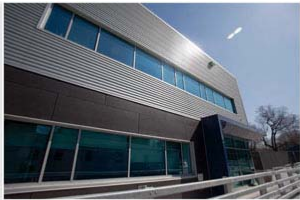
The exterior of the building uses corrugated metal siding.
