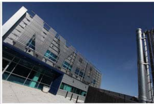
The metal panels of the canopies in the front are painted NYPD blue.
