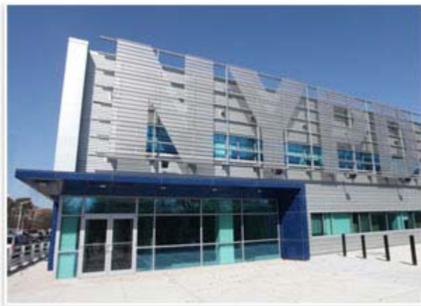
New York City-based Spacesmith's design for the New York City Police Department Tow Pound Operations Building garnered a design award in the office building category from the Brooklyn Chamber of Commerce. The facility opened this spring and is expected to become LEED Gold certified.
