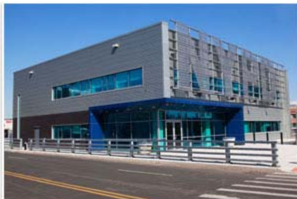
Large NYPD signage on the latticework on the front of the building increases visibility. The perforated stainless steel
